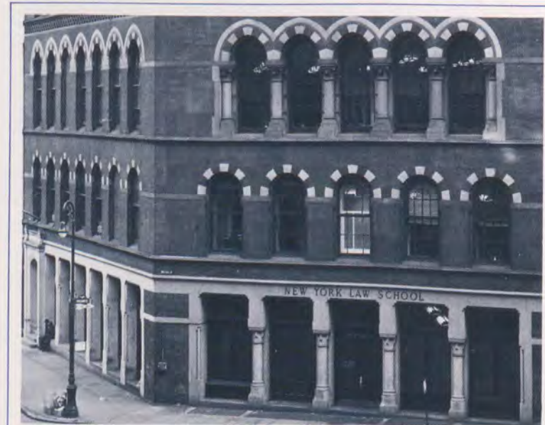
Dwight Building, 244 William Street The Law School's home 1947 – 1962
