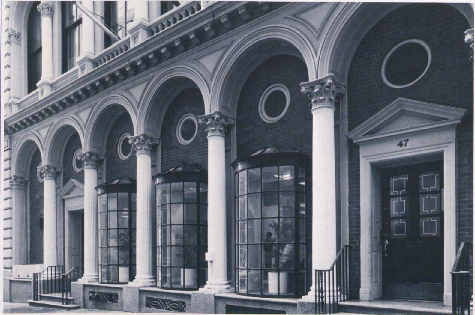
New York Law School's building at 47 Worth Street
