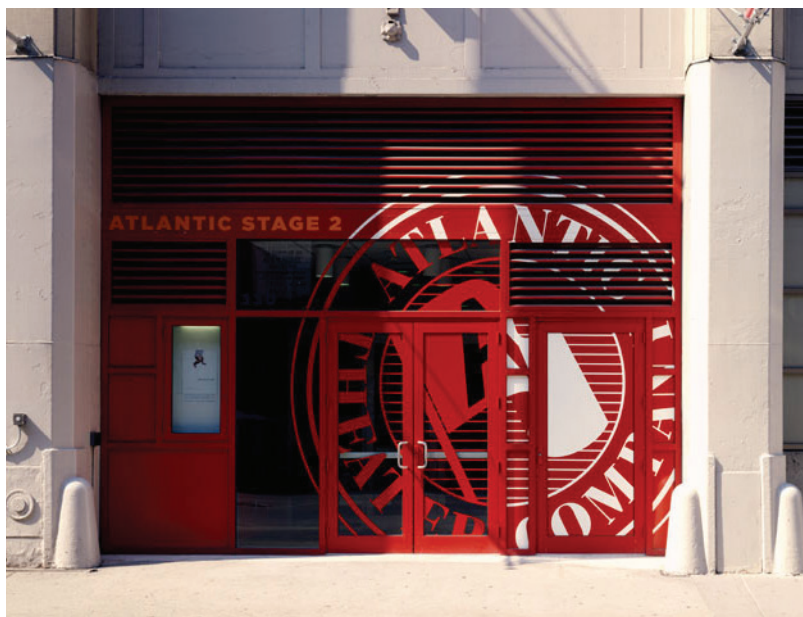
Atlantic Stage 2 (completed, street-level entrance) – Photo by Catherine Tighe
