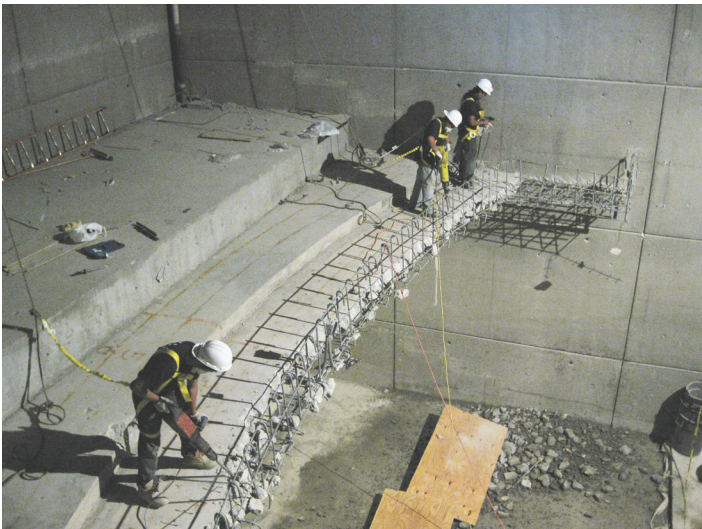
Baryshnikov Arts Center (mid-construction, specifically during removal of the prior balcony) — Courtesy of Denham Wolf
