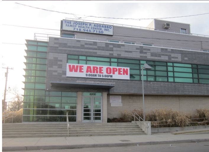
Joseph P. Addabbo Family Health Center (phase 1 completed, photo taken immediately after Sandy) — Courtesy of Denham Wolf
