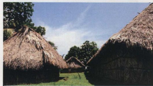
A traditional Garifuna hut made of sugar cane sticks and mud, with no running water or electricity.
